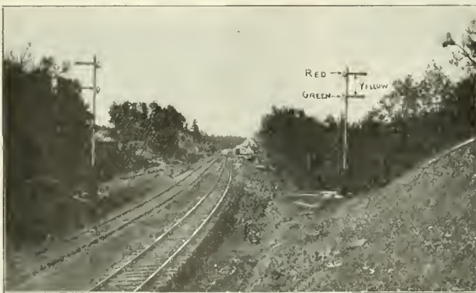
FIG. 10. RIGHT-HAND TRACK; BOTH BLOCKS IN ADVANCE OCCUPIED—STOP.
